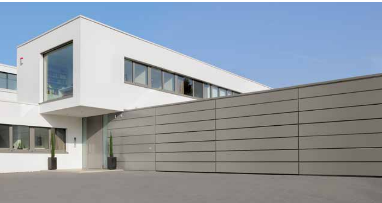
On-site cladding with aluminium compound board
